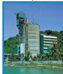
Terminal Lembar, Lombok Lembar Terminal, Lombok
